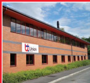
UK Headquarters and Technical Centre
